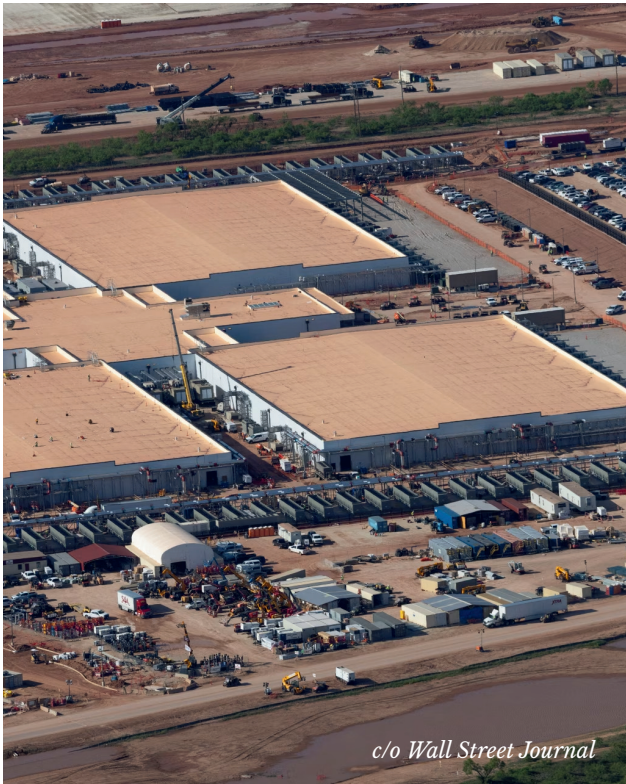
OpenAI's Texas Data Center
